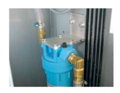
Screw the fine particle filter out of its housing and replace it.
