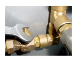
Screw the coarse filter out of its brass housing using the open-ended spanner (SW 20) and clean it with compressed air. The filter is located underneath the service unit.
