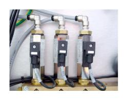
Check the correct setting of the flow monitor. Compare it with the IBS report.
