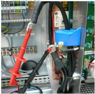
4. Measure the resistant of booth cable to earth. If the value is very low maybe the transformer primary side have short circuit to earth or the cables are damaged and make some contact to earth. If looks ok (endless or very high resistant) go to point 5.
